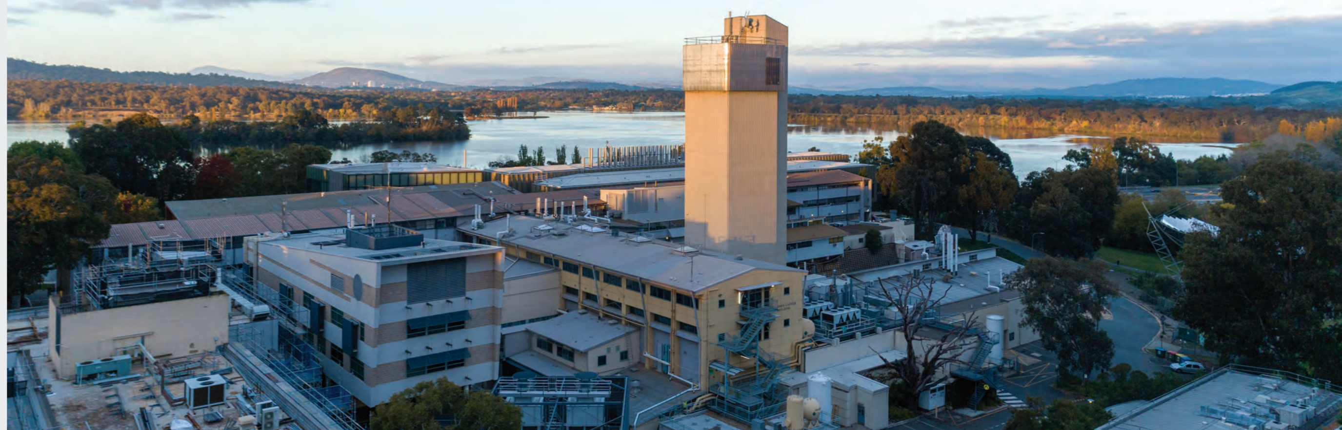
The Heavy Ion Accelerator Facility towers over the ANU Research School of Physics.
